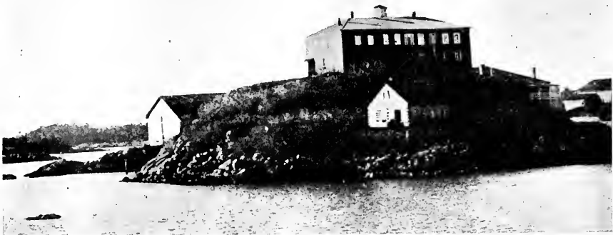
Baranof Castle, the Russian Governor's headquarters, was built of square timbers and fastened throughout with copper rods bolted to the rock foundations, the first castle having been overthrown by an earthquake. The building was erected in 1827 and burned to the ground in 1894. In the cupola on the roof a lamp was kept burning, the first lighthouse on the Coast.
